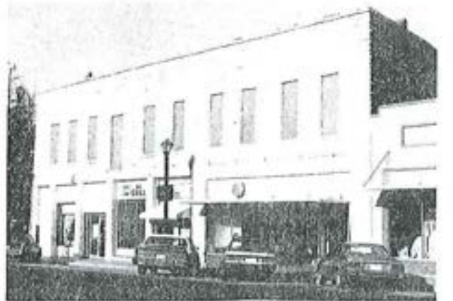
Granite Hotel on S. Broad Street.
