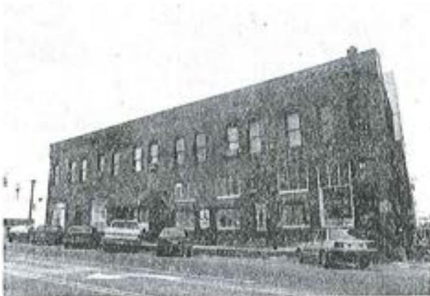
Garrison Building on S. Broad Street.
