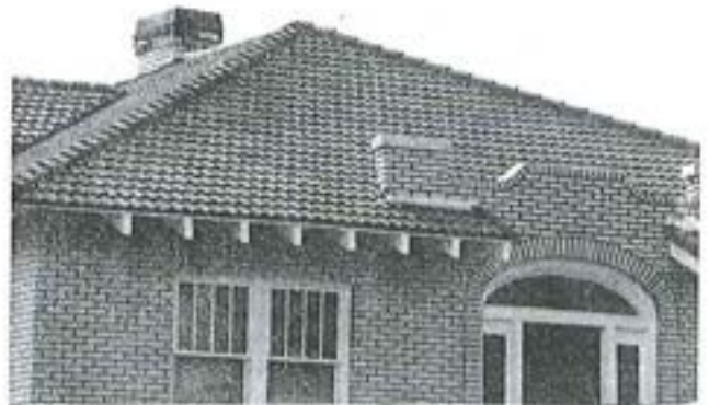
Spanish Mission style tile roof at 217 W. Candler Street.
