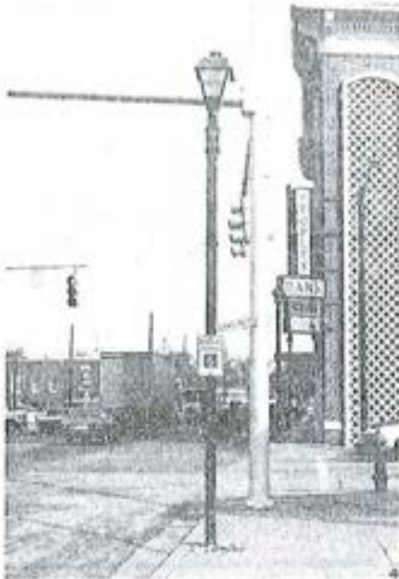
View of Broad Street showing present lighting fixtures.
