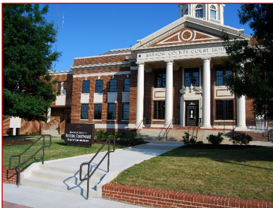
Historic Courthouse Renovation
