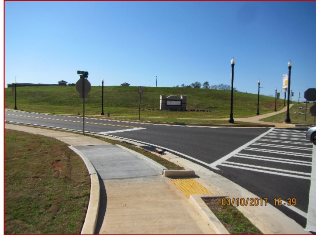
McNeal Road Pedestrian Improvements adjacent to new Barrow County Schools
